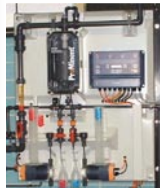
Desinfection of the bottle neck finish with ClO 2 treated water
